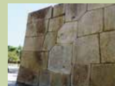
Cut-insertion masonry with porphyritic granite
