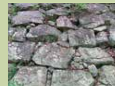
Pound-insertion masonry with sandstone
