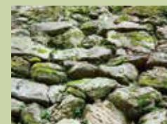
Natural-face masonry with crystalline schist
