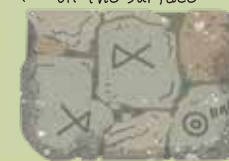
Cut-insertion masonry with porphyritic granite
